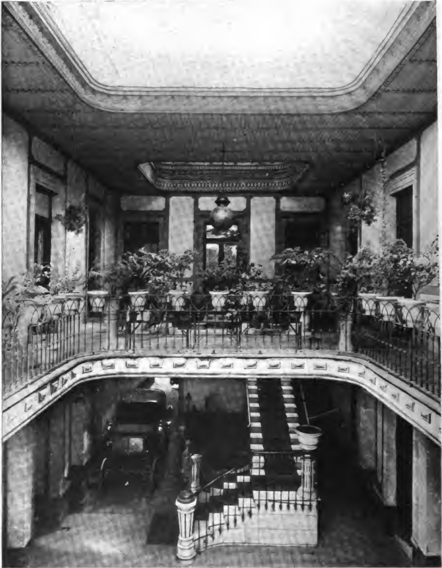
Patio and Corridor.
